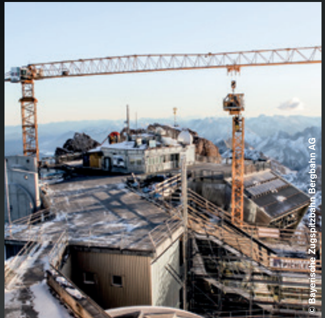
In the drive of the new Zugspitze cableway in Germany.
