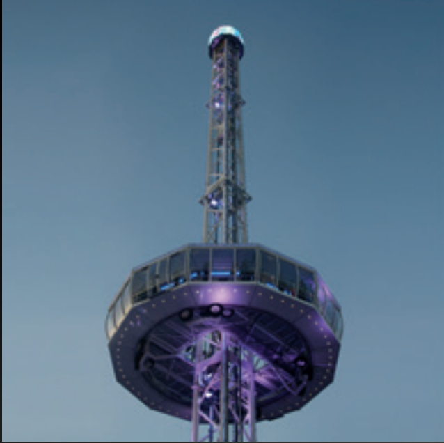
In the drives of the mobile panoramic tower City Skyriser in the Netherlands.
