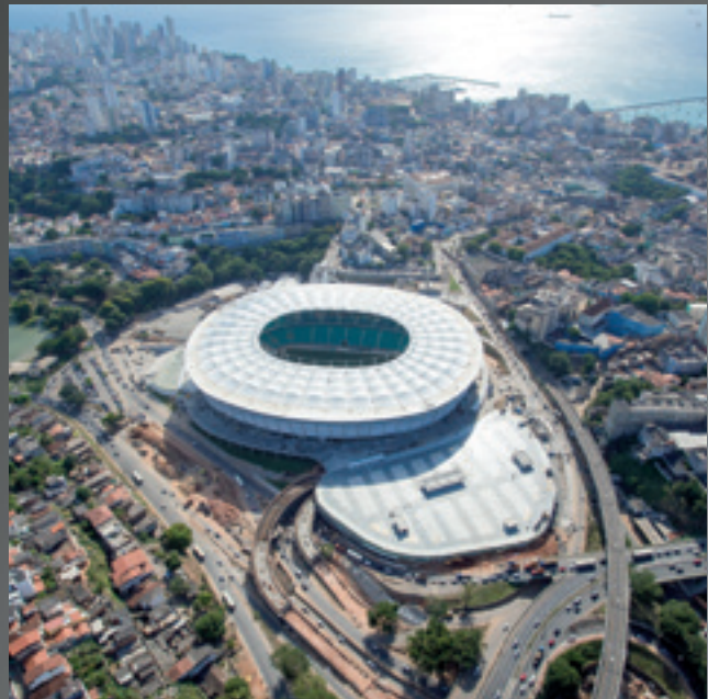
In the concrete pumps for building the access roads to the stadiums of the Soccer World Cup in Brazil.
